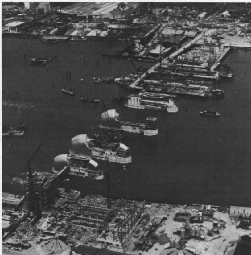
● The Thames barrier being built at Woolwich
