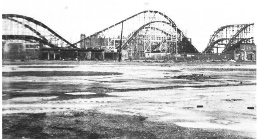
● Coney Island - "turned off by crime and decay, tourists stayed away".
