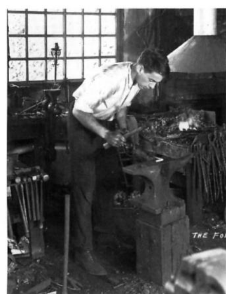
In heyday, Arden Forge made fine ironwork, such as andirons, sconces.
