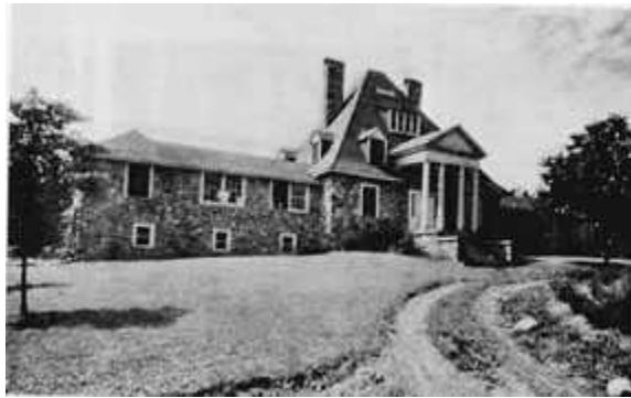
"Dogwoods," the Main House on the Homestead. One of the Wings Contains the Workshop, the Other, the Loom Room. Designed and Built by Amateur Labor. Even the Wiring, Plumbing, and Steamfitting Were Done by What Can at Best be Described as Semi-skilled Labor. The Stonework in All the Houses on "Dogwoods" Was Put in by Amateurs, Using a Modification of the Flagg Method of Wall-building.
