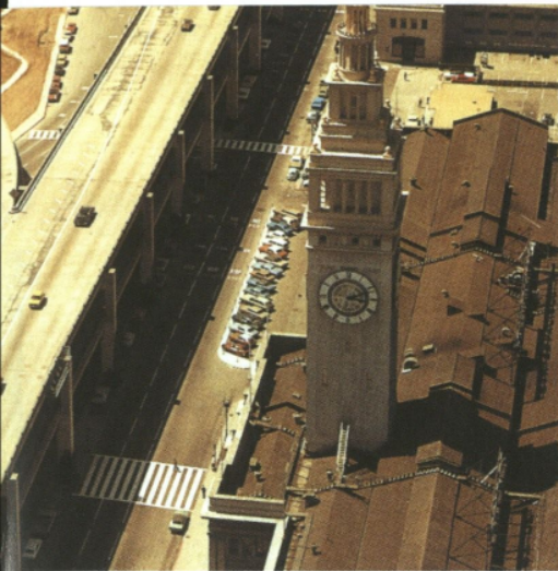
ed growth. Demolition and sealions (below left) changed that
