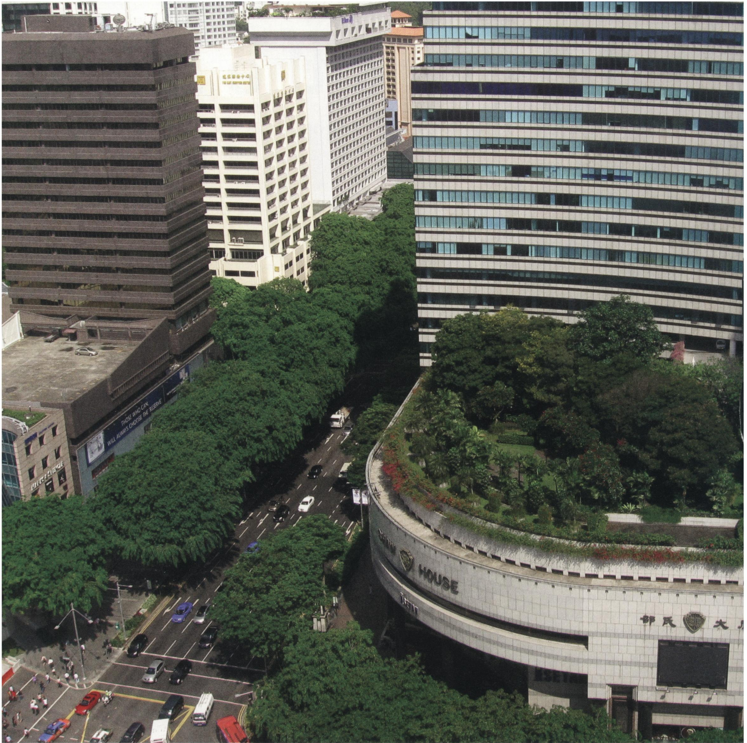
Green roofs like this one in Singapore's central business district capture rainwater to help lessen the effects of stormwater on sewer systems.
